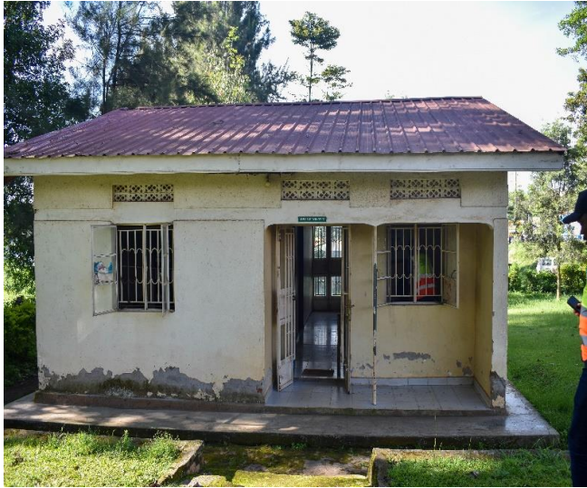
Itwara Forest Sector Office to be renovated
