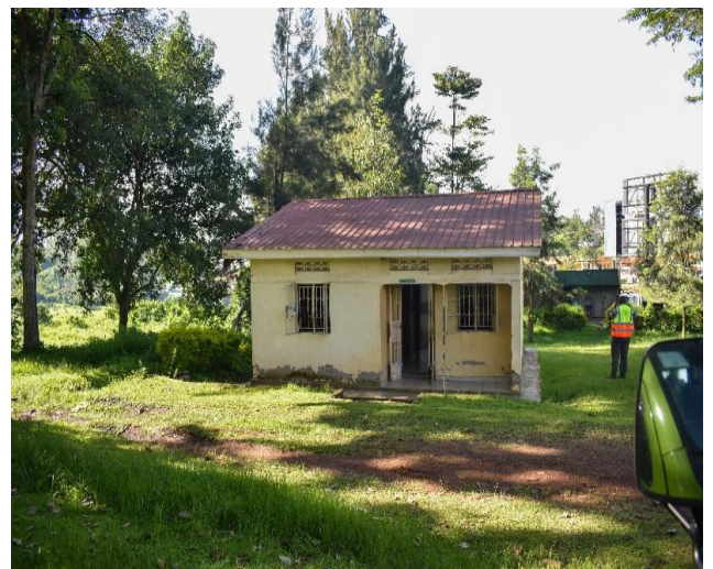
Pathway cutting through Itwara Sector Office
